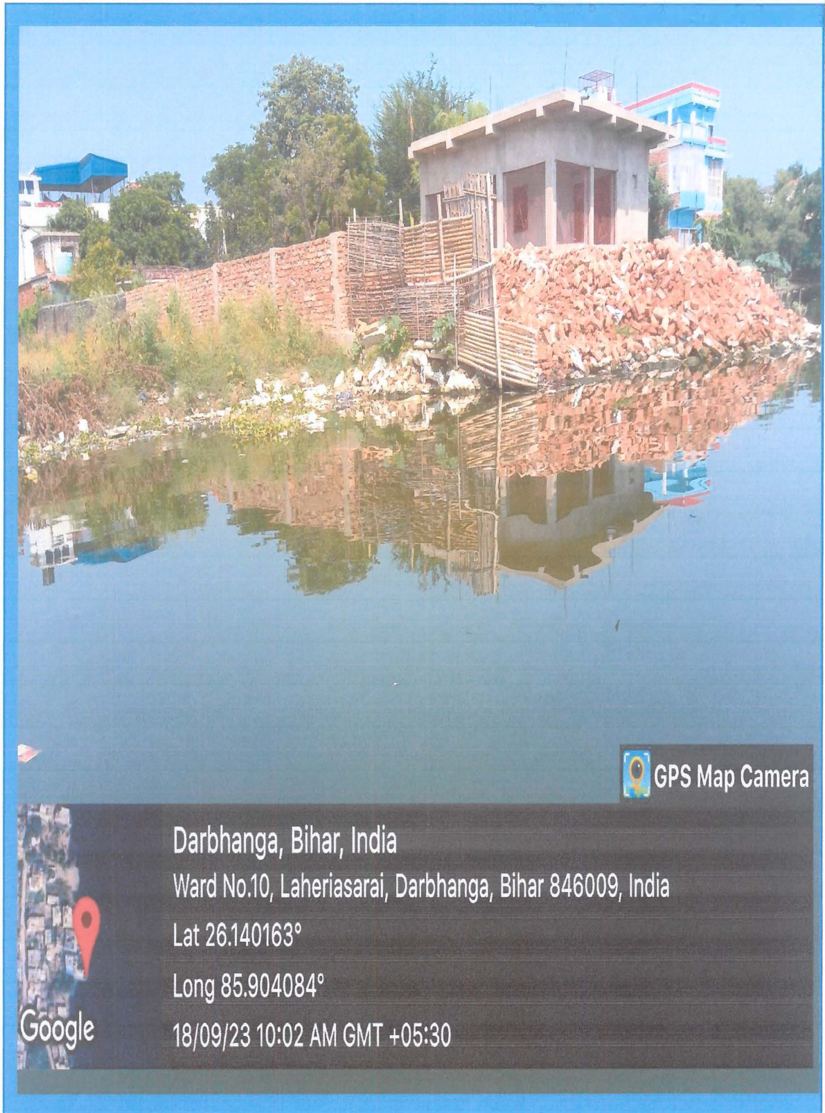
Photo No. 7, Ganga Sagar Lake, Fresh Encroachment
